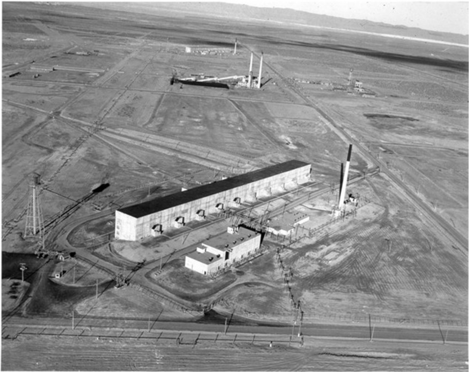
T Plant . Photo credit: Department of Energy
